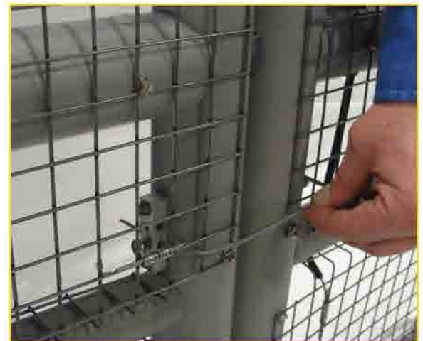
Run jumper wire to adjacent panel
