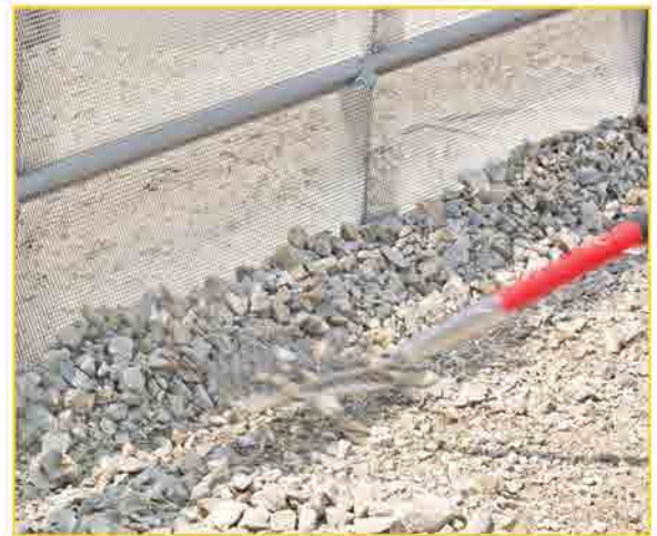
Rake gravel on inside and outside of bottom rail of connecting panels
